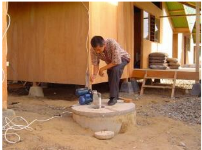
Elder Subandriyo examines one of 7 wells with pumps that provide basic water supply for homes
