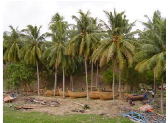
Construction yard for 10-meter boats
