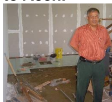
Sutarno helping rebuild a facility at IAIN Islamic Studies University
