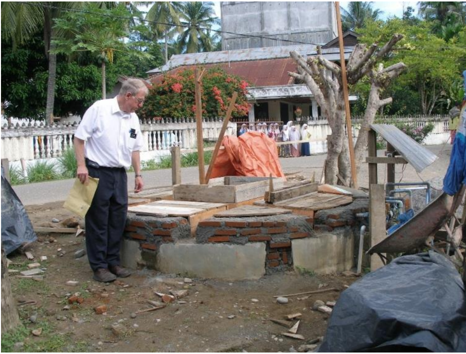
Well covering under construction
