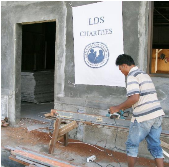
Construction worker working on the renovation of the old building.
