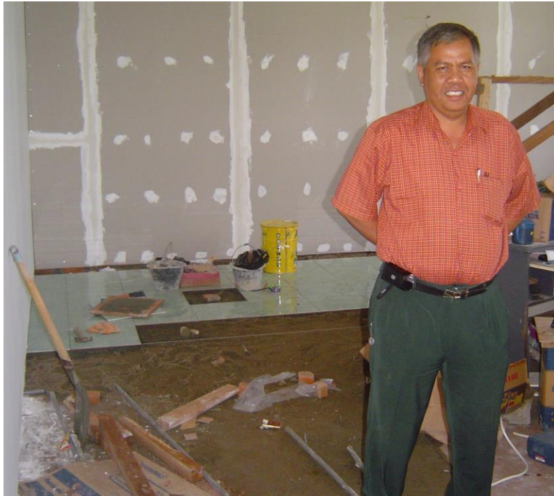
Sutarno remodeling a room to assist with Computer Lab improvements
