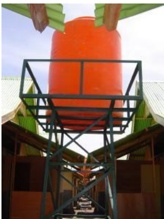
Water storage tanks store water from wells and provide for 4 homes each
