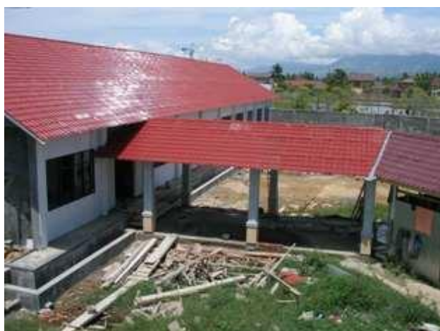
Vocational rehabilitation building under construction.
