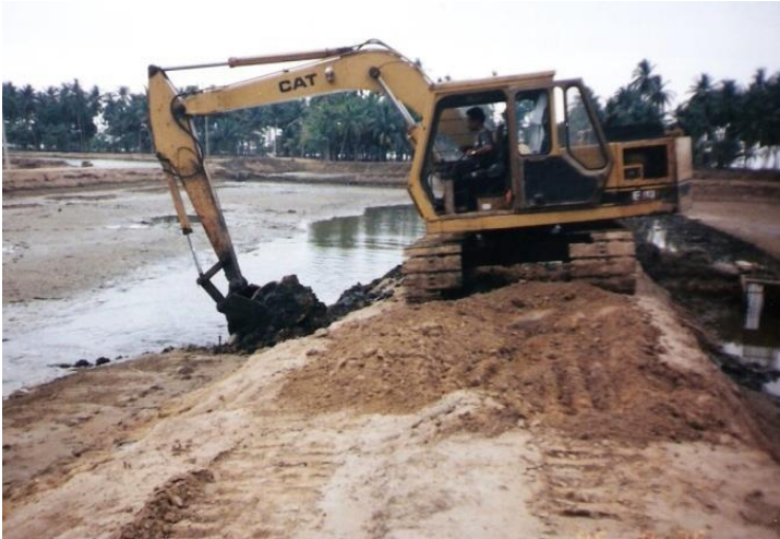
Backhoe shaping shrimp/fish pond banks
