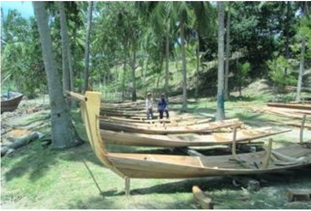
Construction in boat yard at Krueng Raya
