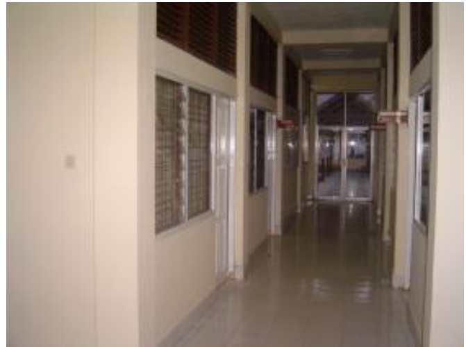
Mental Hospital condition after paint and upgrades
