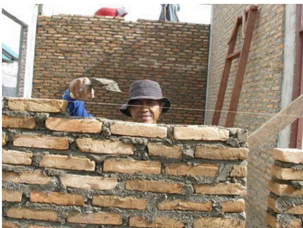
Brick layer working on vocational rehabilitation building
