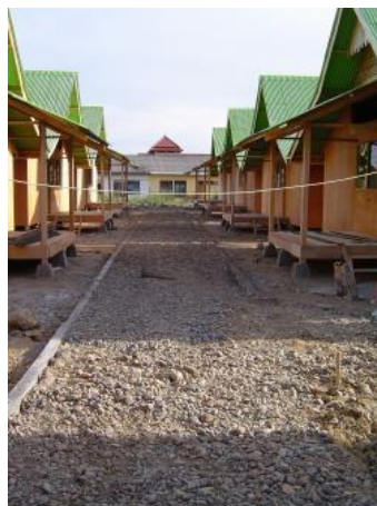
Gravel pathways were added due to extreme muddy conditions following the rains
