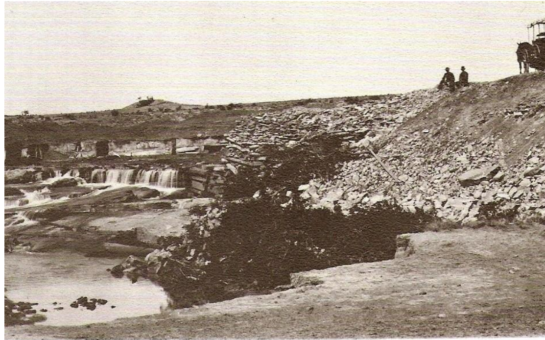
The 8th earth-fill diversion dam built on the Little Colorado River by Mormon pioneers of St. Joseph, Ariz. It was begun in March, 1891 and is shown after completion on 10 March 1894. The natural rock spillway is at the left.
