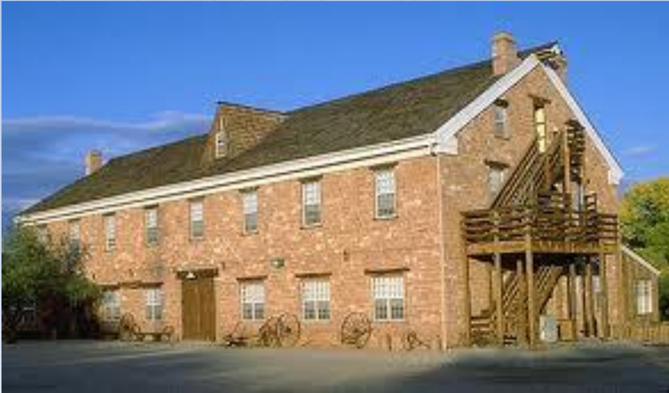
Santa Clara Fort (walls were three feet thick)
