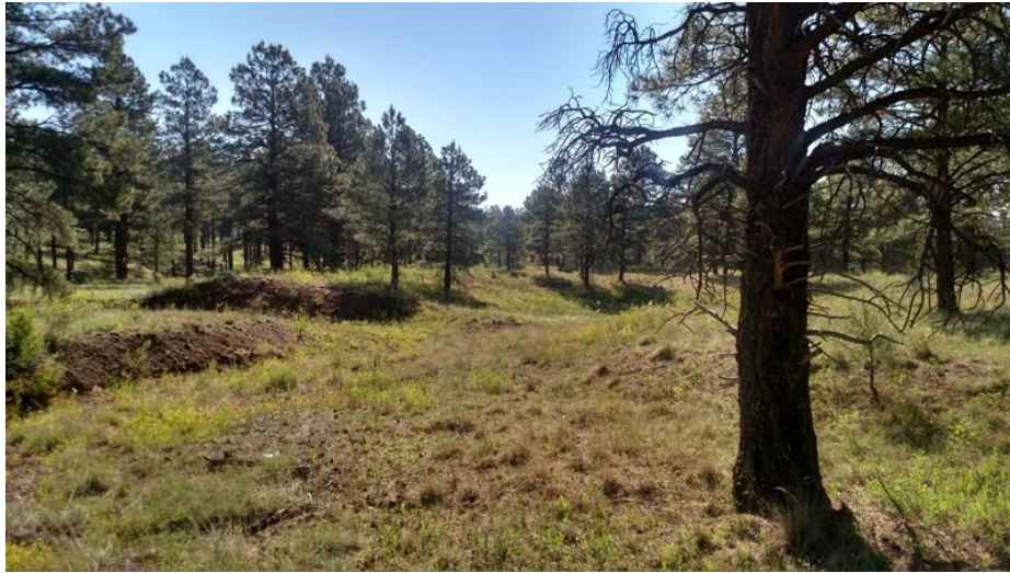
This Dirt Tank just downstream from rock dam provides a small retention basin to catch overflow from the rock dam
