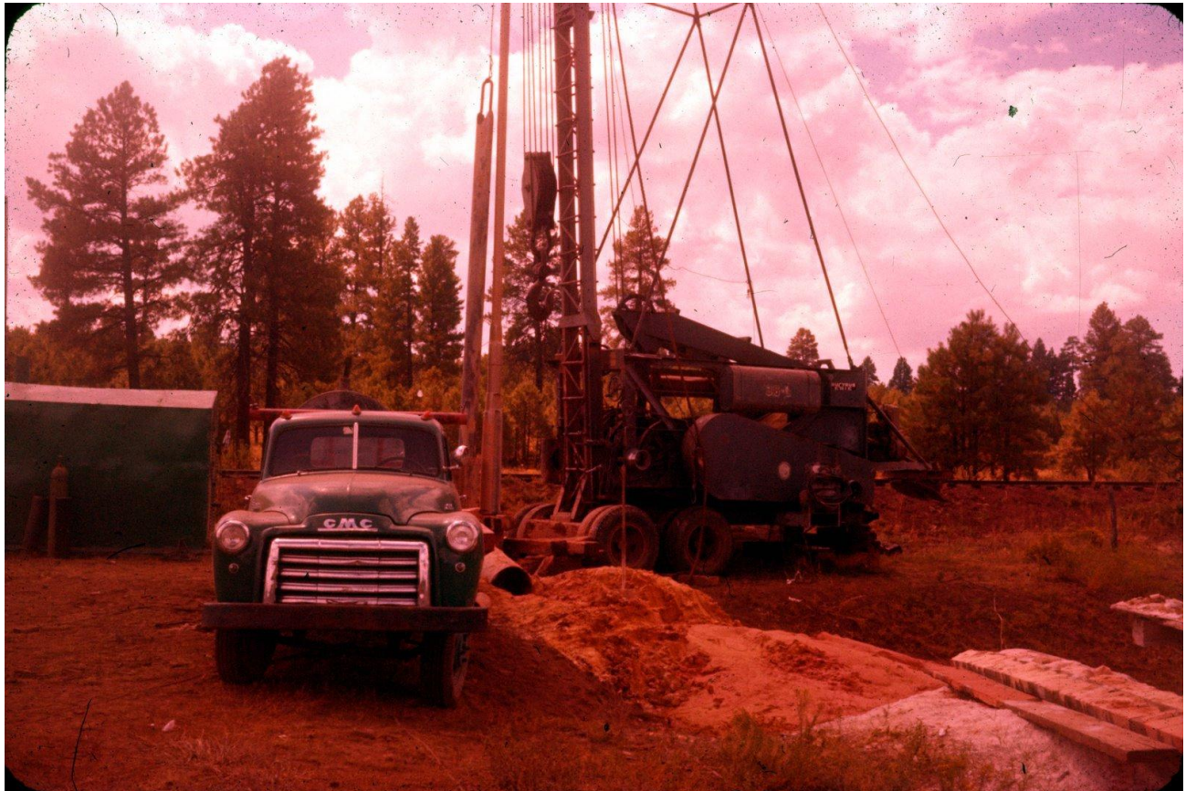
Drilling of first well with railroad in background
