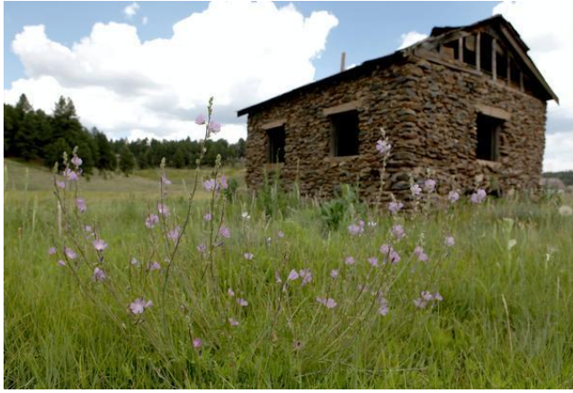
Pump House facility at Kachina Village
