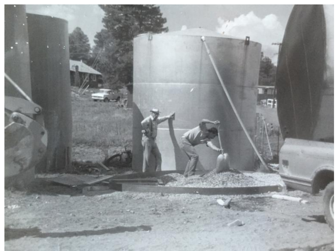
Nick leveling gravel to install a new 10,000 gallon water storage tank.
